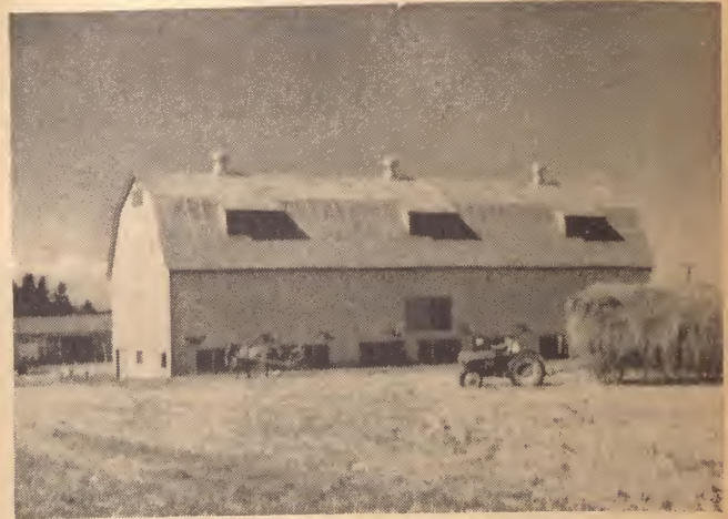
The new 108 x 38 barn on Ralph Zwicker's farm.
